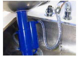
Flush condenser via tube
