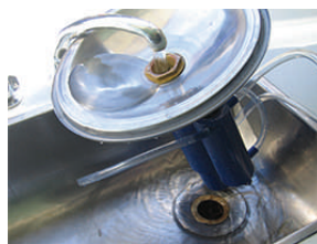
Flush column and packing
