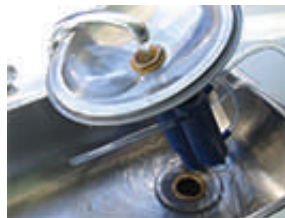
Flush column and packing
